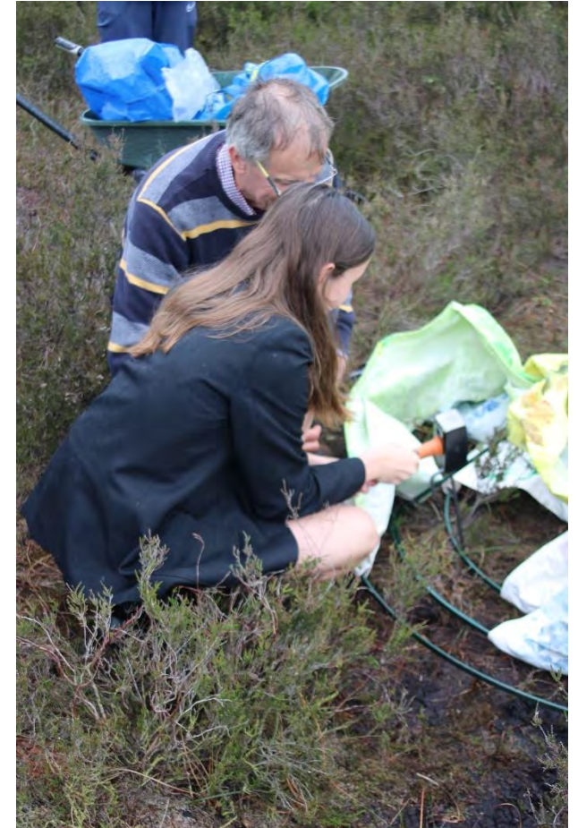
Installation in progress
